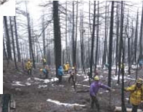
Log erosion barriers near Lemon Dam
